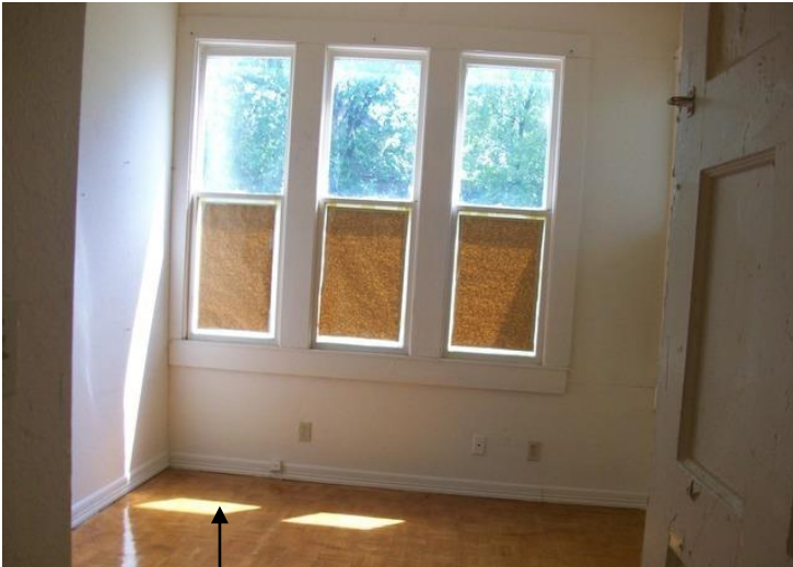
New subflooring and flooring needed (Warped and shifted)
